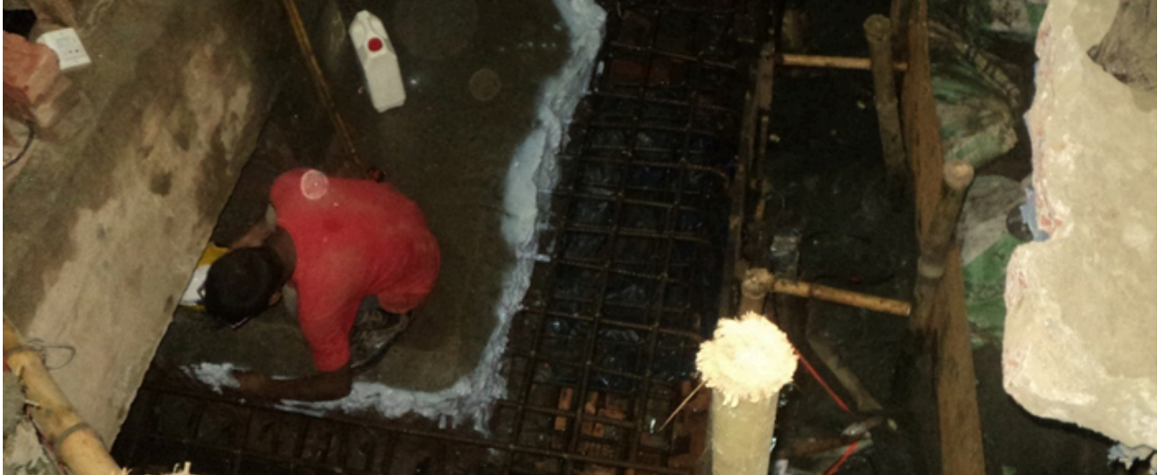
Picture no. 7.1: Footing retrofitting works
