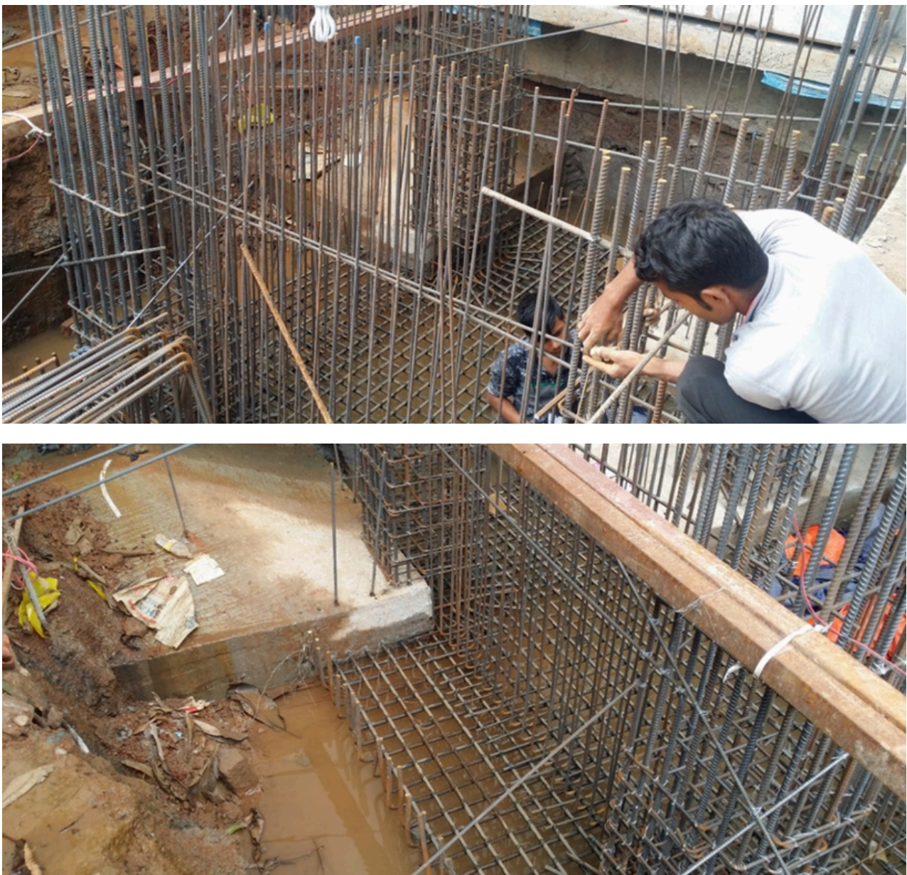
Picture no. 1.1: External Steel Lift framing foundation construction
