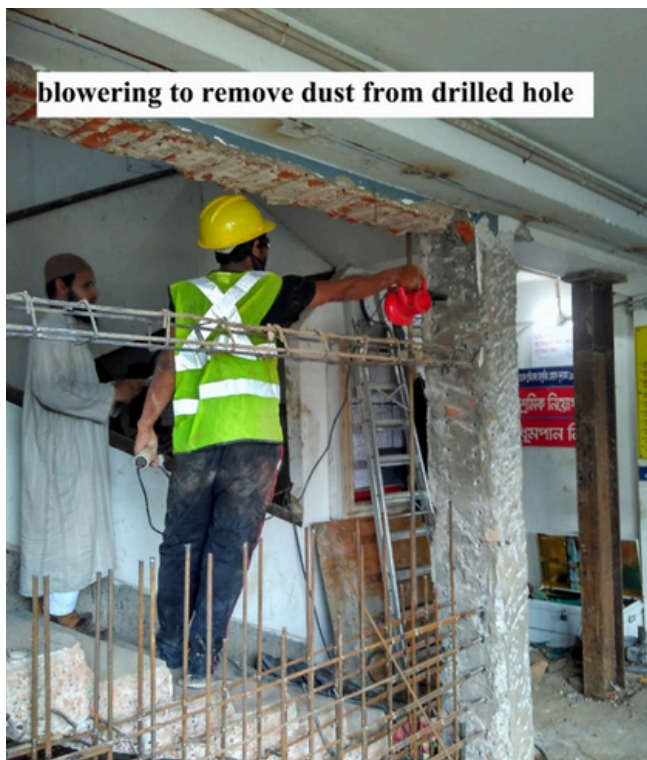
Picture no. 8.2: Shear wall construction works in existing building
