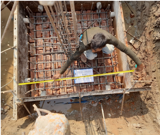
Picture no. 5.1: Foundation size inspection
