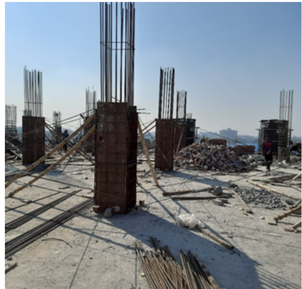
Picture no. 4.4: Steel Shuttering for column casting
