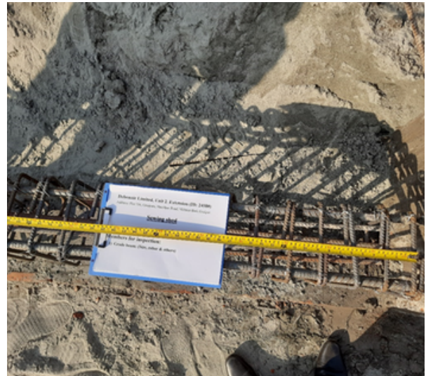
Picture no. 5.2: Grade beam stirrup spacing check
