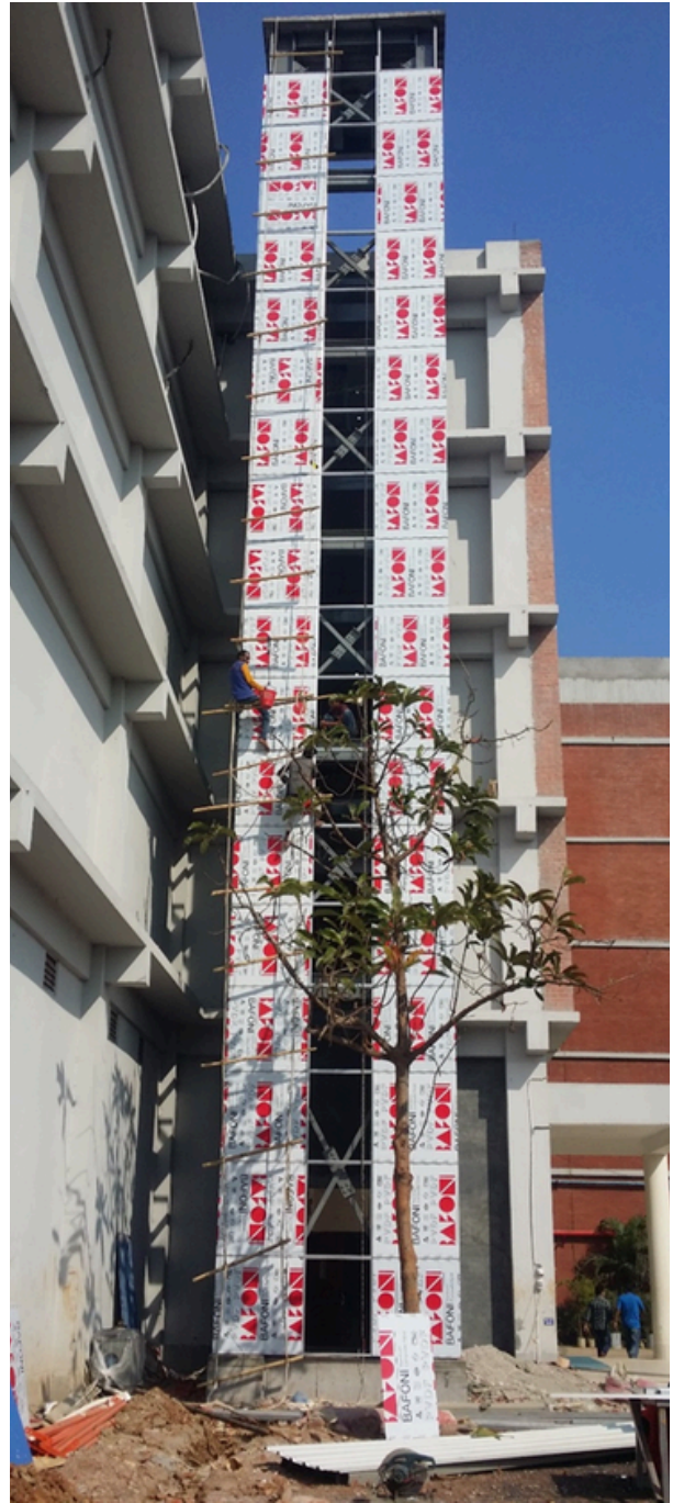
Picture no. 1.2: External Steel Lift framing construction works
