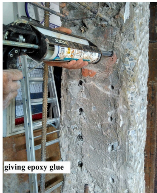
Picture no. 8.2: Shear wall construction works in existing building
