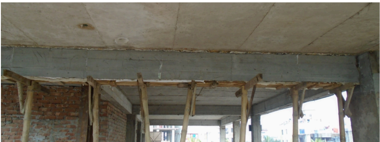
Picture no. 7.5: Beam retrofitting works completed
