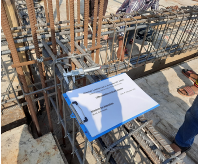
Picture no. 4.1: Beam reinforcement dia check
