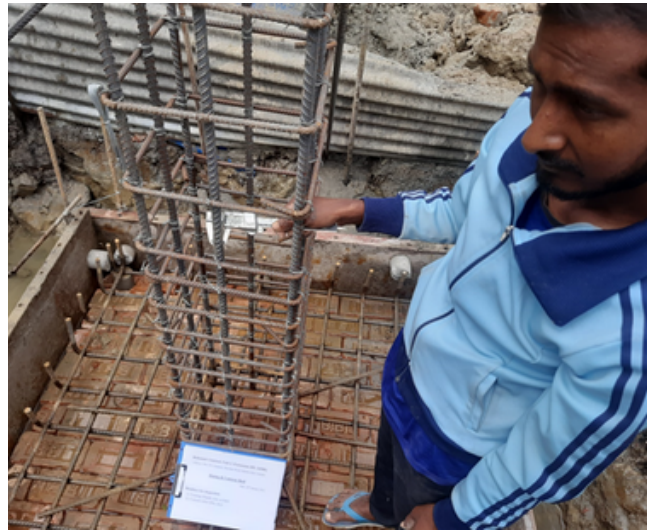
Picture no. 3.2: Column Tie dia inspection
