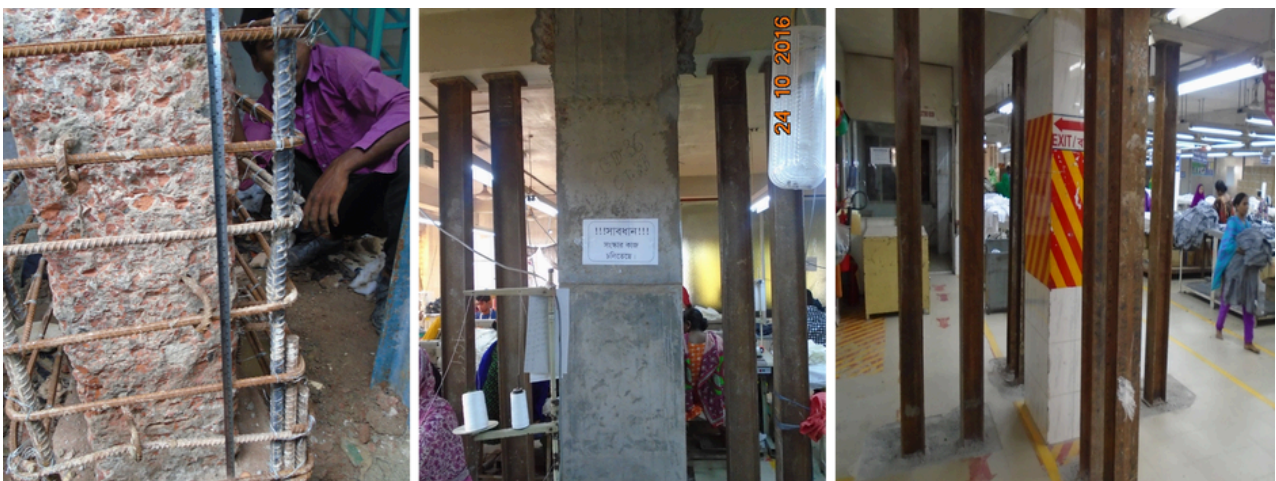
Picture no. 7.3: Column retrofitting works
