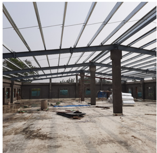
Picture no. 5.4: Rafter & Purlin setup going on
