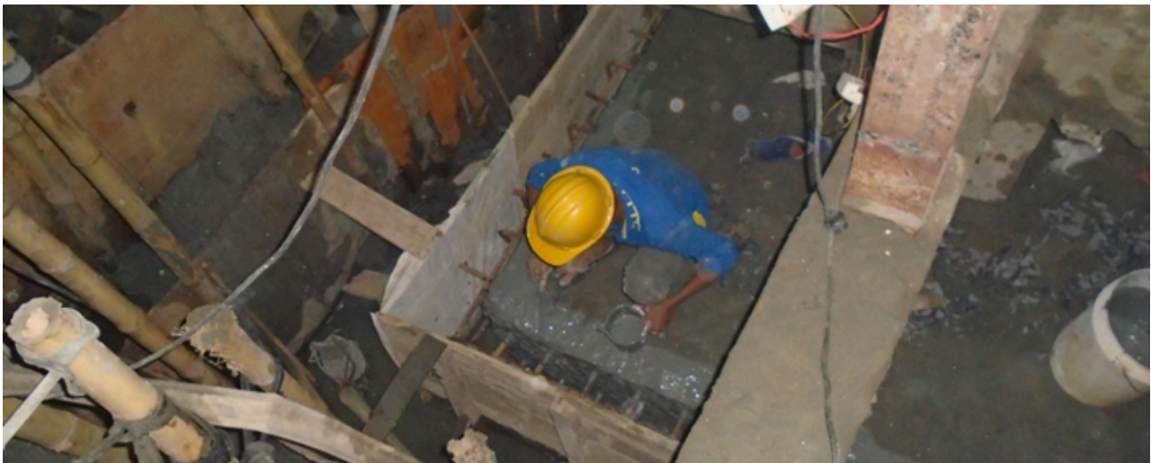
Picture no. 7.2: Footing retrofitting works
