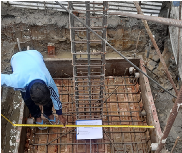
Picture no. 3.1: Foundation size inspection
