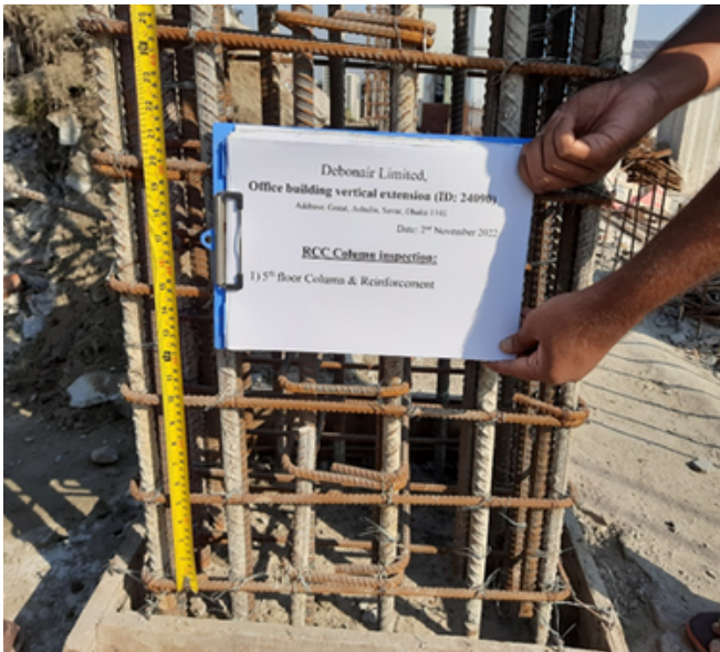
Picture no. 4.3: Tie bar spacing checking (at 5th floor)
