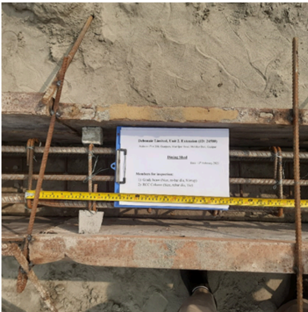
Picture no. 3.3: Grade beam stirrup spacing check
