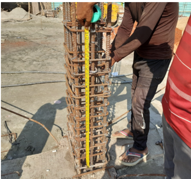
Picture no. 5.3: Column tie spacing check
