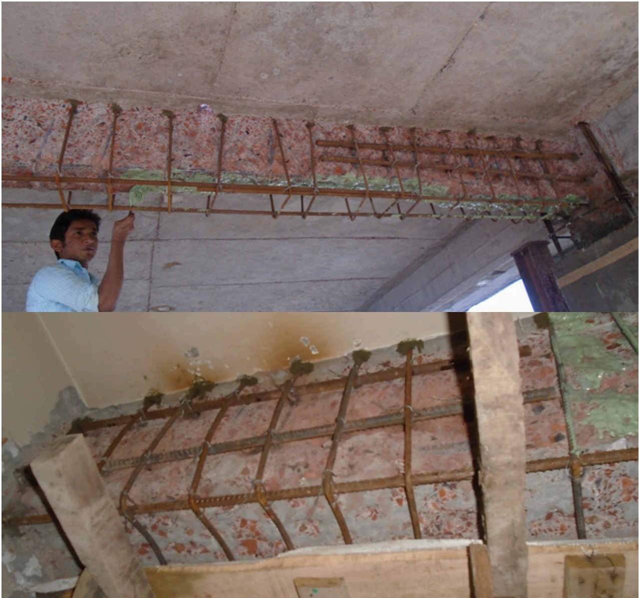
Picture no. 7.4: Beam retrofitting works going on
