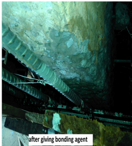
Picture no. 8.1: Column jacketing works
