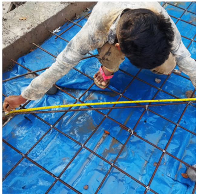
Picture no. 3.4: Hair pin rebar at floor slab
